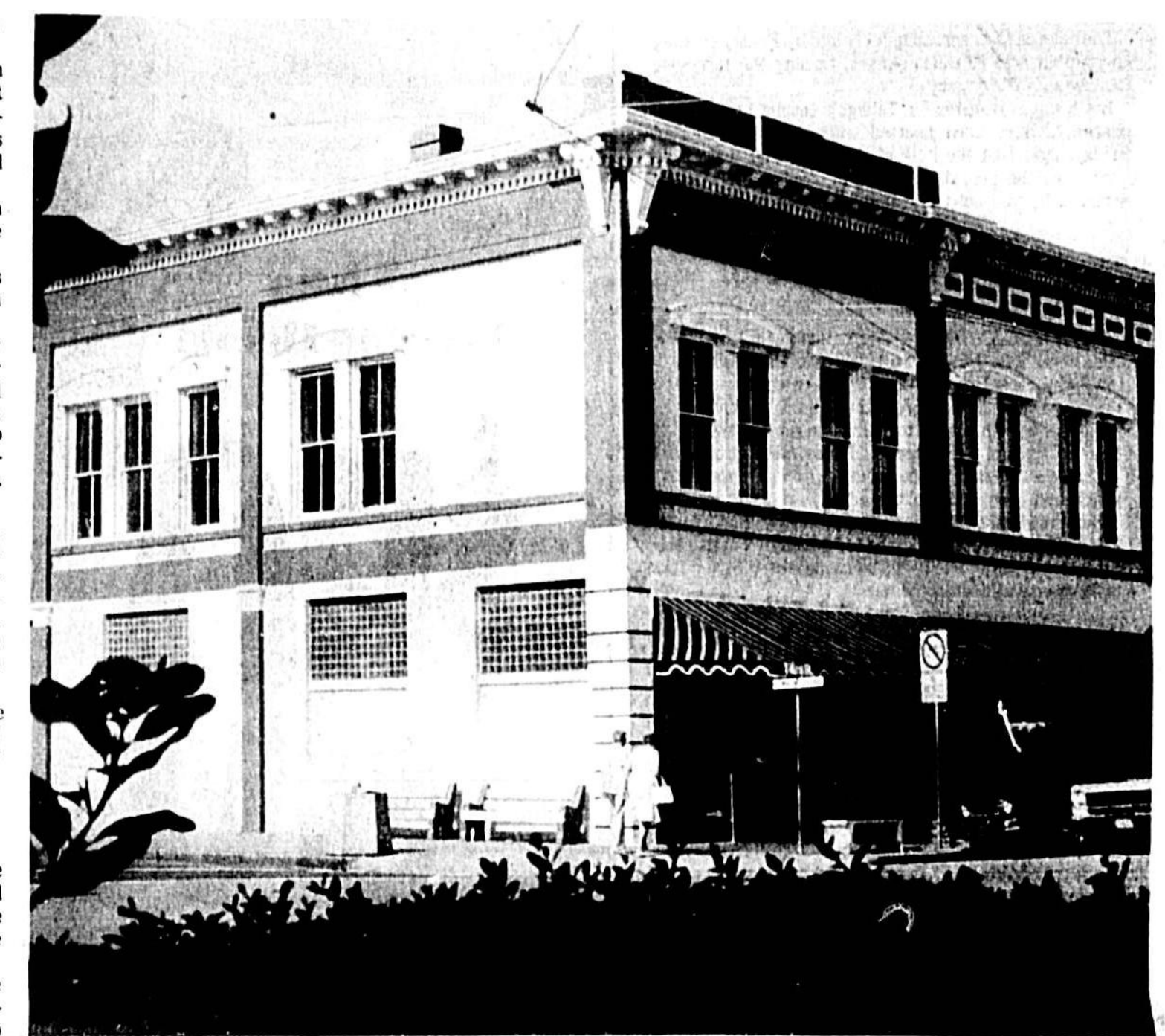
The proprietors of Touchton's Rexall Drug Co., at 121 E. First St., Sanford, were among the downtown businessmen who demonstrated their commitment to the business district renovation project by overhauling the outside appearance of their building. Now it's the commission's turn to determine how much the city will invest in the image-building program.
