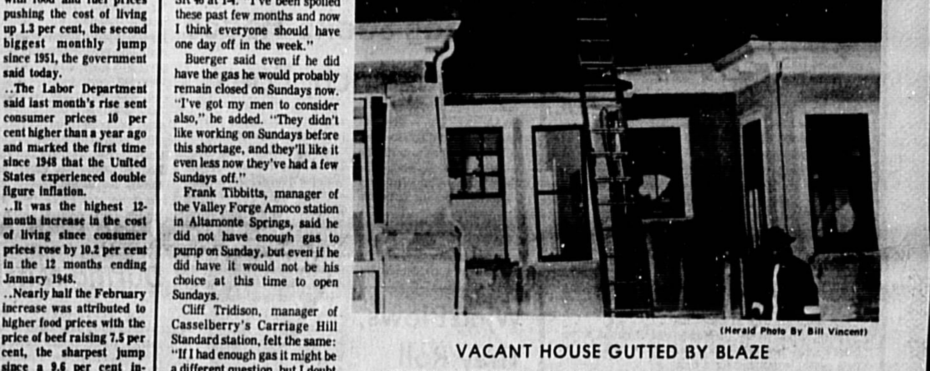
SANFORD FIREMEN battled flames for two hours this morning at 119 Elm Avenue, Sanford, Fire Chief G. M. Harriett said. The house has been condemned by the city and the owner is unknown. Firemen said the blaze may have resulted from a dropped cigarette. City condemned house because it was abandoned.
