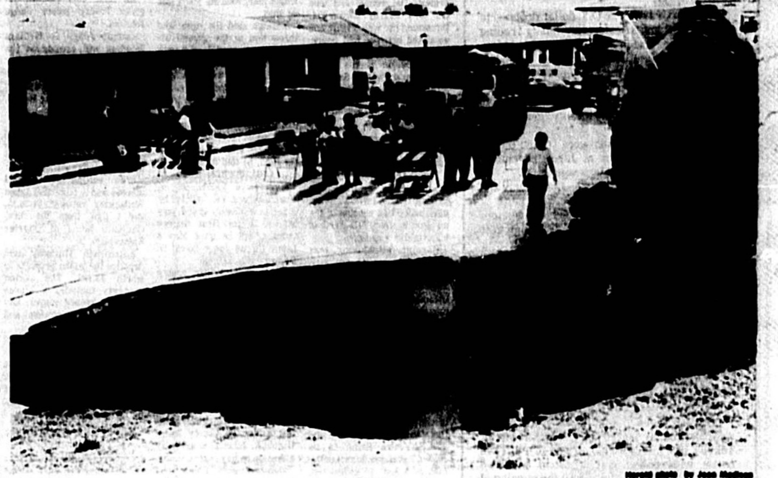
THE SINKHOLE AT APARTMENT COMPLEX ON PALM SPRINGS ROAD NEAR 638
