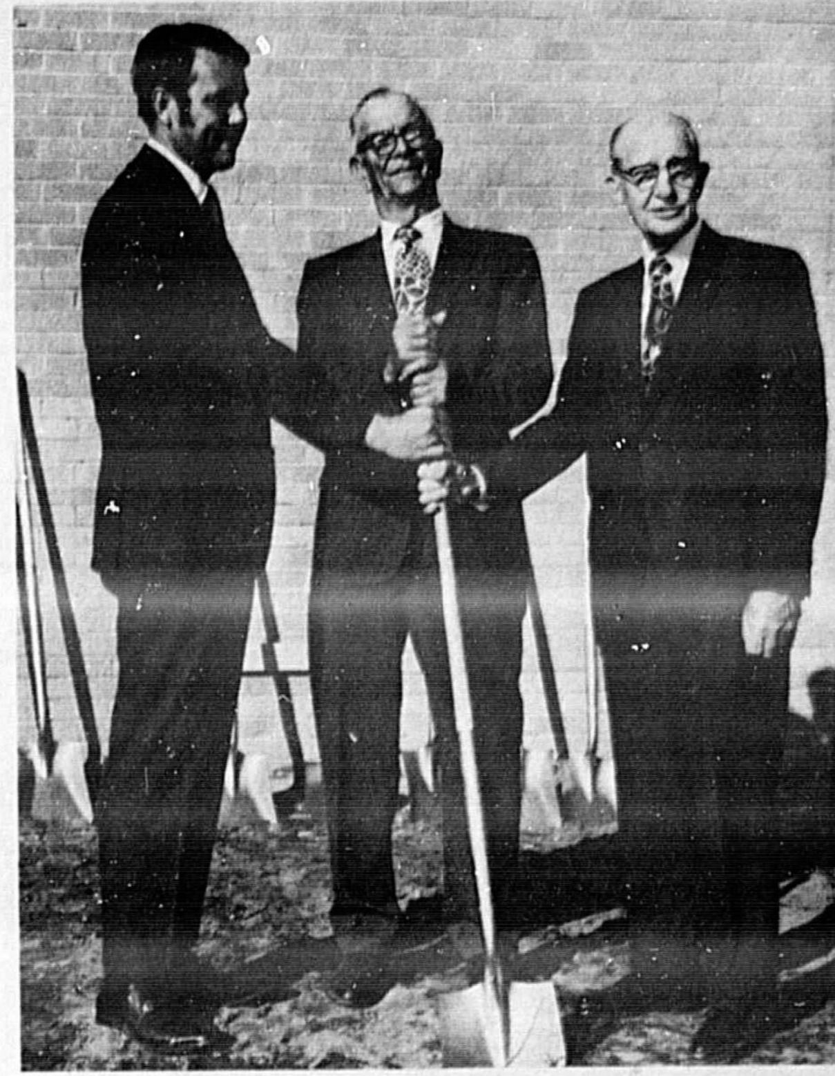
HIGH HOPES Official groundbreaking was held this morning for the new million dollar-plus high-rise addition to First Federal Savings and Loan of Seminole County's First Street facility. Left to right, Gib Edmonds, executive vice president; E. C. Harper Sr., president; and George Touhy, director. (Staff Photo)
