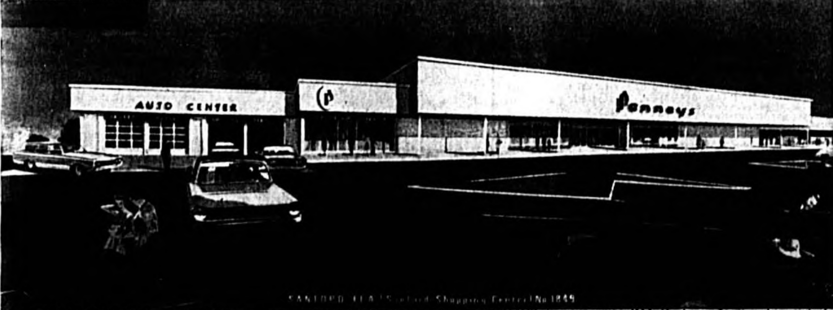
EXEMPLIFYING the "new look" in Penney operations throughout the nation is the company's new Sanford Plaza store, (shown in the artist's rendering), which will open later
