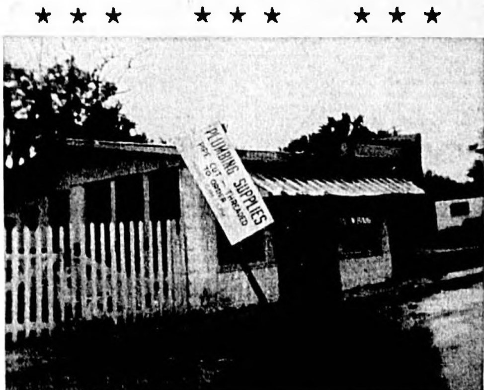
HURRICANE FORCE WINDS ripped off the sign and part of the roof at George Reek and Son Plumbing on E. Lake Ave. in Longwood during this morning's wind and rain storm onslaught which hit the entire South Seminole area. Damages were estimated at some $200 to the building. (Herald Photo)
