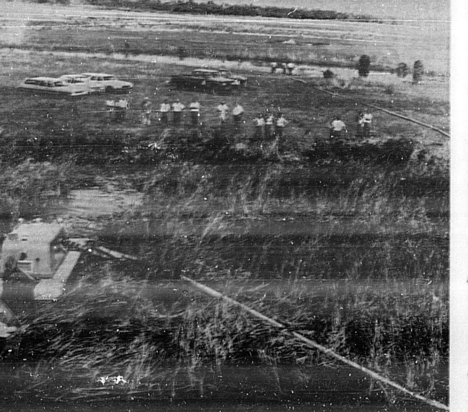
A "MUDCAT" was demonstrated Wednesday afternoon for State Game and Fresh Water Fish Commission officials at Lake Golden. The device, manufactured by Inland Service, of Minneapolis and Sanford Airport, clears weeds and debris from the beds of lakes and waterways, carrying the refuse in a pipe (lower right and center right) to a dumping spot. (Bill Vincent Jr. Aerial Photo)
