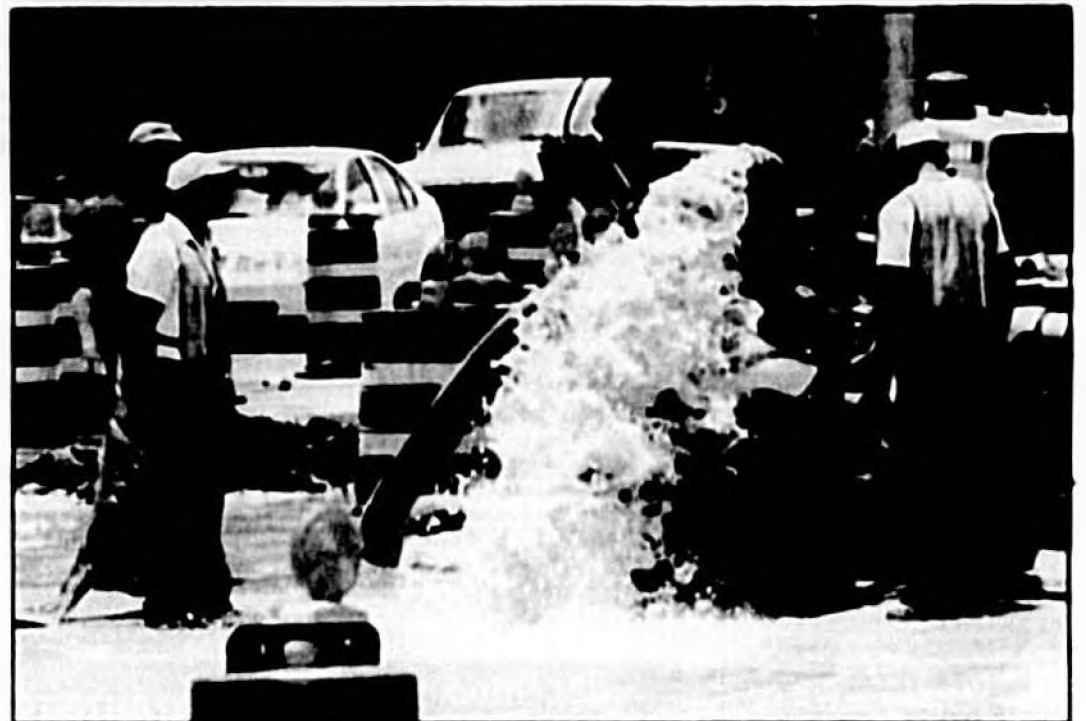
Sanford utility department workers attempt to repair a water main break on Airport Road near 25th Street. The break occurred as workers tried to switch from the old 24-inch line to a newly installed line. Nearly all Sanford residents experienced substantially reduced water pressure, and a citywide boil water alert was issued and will may continue until at least Thursday evening.
