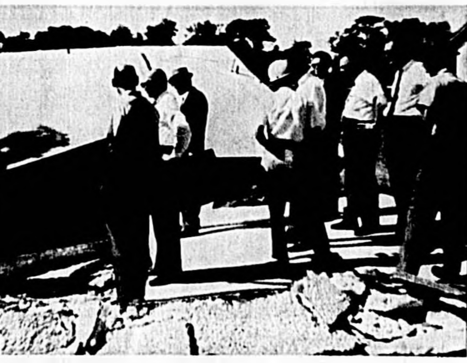
STATE, COUNTY and Casselberry officials survey the ruins of the Richard Rozolsky home which dropped 12-14 feet into a sinkhole on Northmoor Road at Casselberry Saturday. Gov. Haydon Burns has ordered all-out assistance to the city. (Herald Photo)
