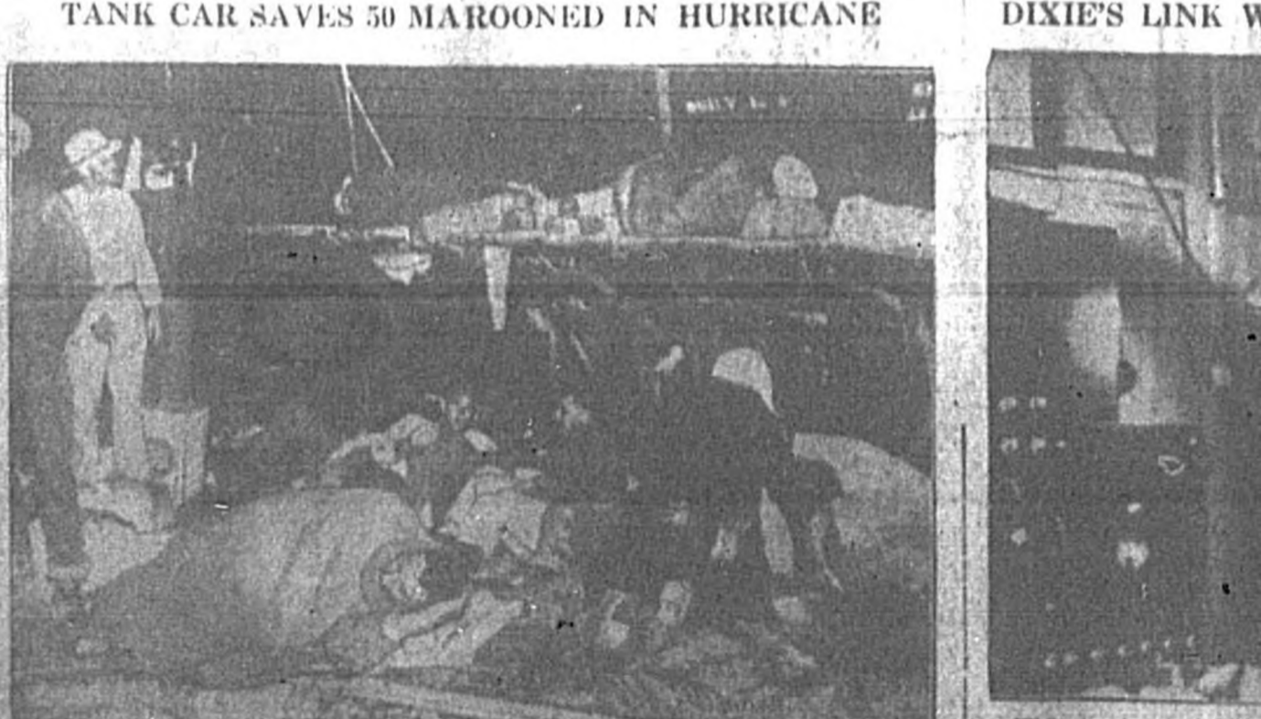
When the West Indies hurricane struck Upper Matecumbe Key, spreading death and destruction, a tank car saved 50 marooned men by being blown to a safe place. The workers were trapped in the building, but they were saved by the tank car. (Associated Press Photo)
