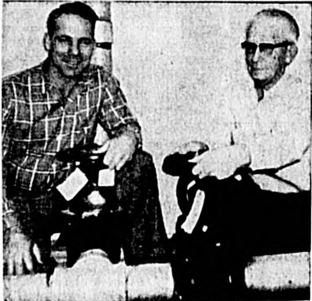
FIRST WATER SYSTEM in the history of Oviedo went into operation early this month at Mead Manor. Opening the valves were Mayor Lee Gary, right and Ben Ward, president of Oviedo Land Company, developers of the new residential area. Owned by Central Florida Utilities, the new system cost approximately $33,000 and will supply 90 homes. (Herald Photo)
