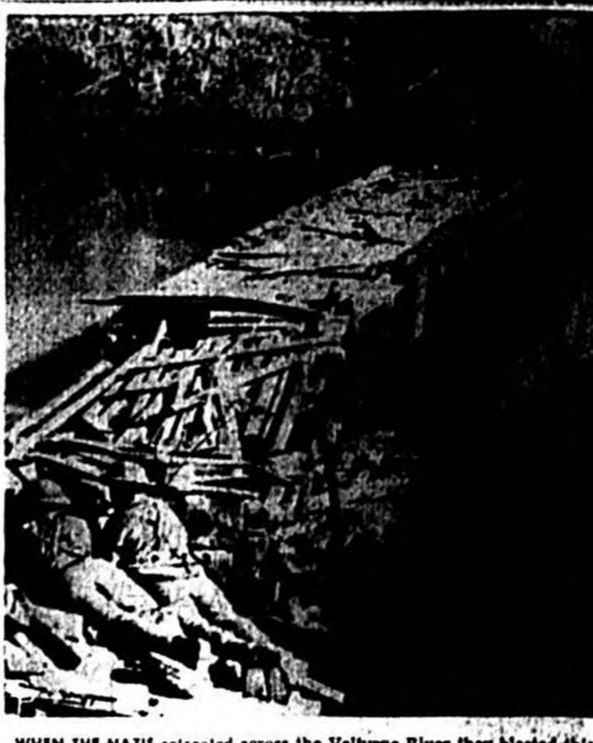
WHEN THE NAZIS retreated across the Volturno River they blasted this small bridge. Ten British soldiers attached to the Fifth Army were engaged in repairing a larger bridge within enemy gun range further along the river. (International)
