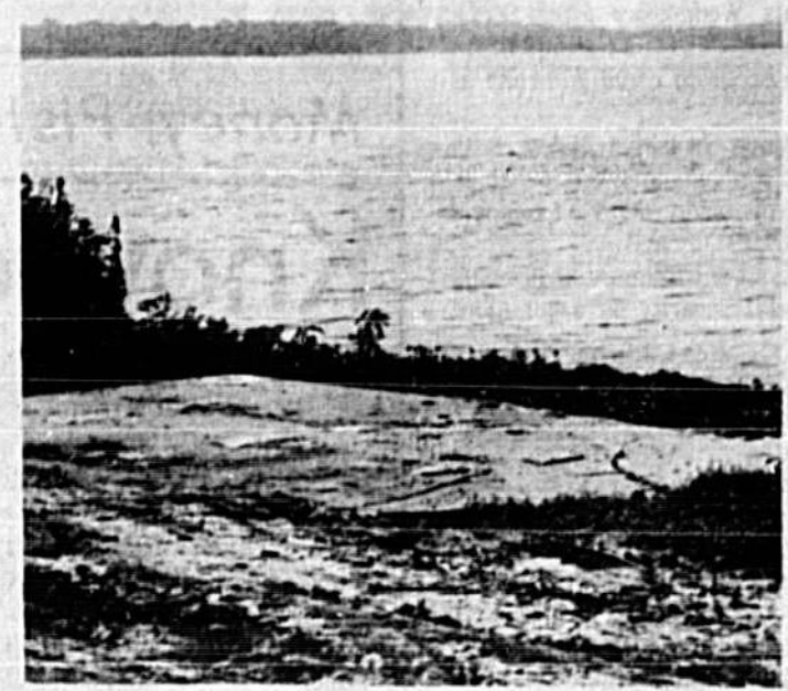
This concrete slab used to be a wayside park overlooking Lake Monroe — before the Florida Department of Transportation tore down the picnic table and shelter this week.
