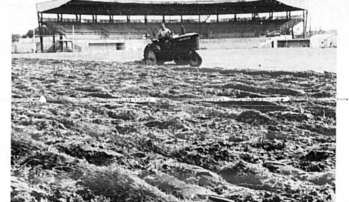
RENOVATION OF THE Sanford Stadium is currently underway by the Seminole High Booster's Club. Here, the field is being plowed in preparation for new sod which will be put in. The school board had excluded $50,000 for new lights at the stadium, which was promised earlier, but are studying costs of upgrading the present lights. (Joe Bush Photo)
