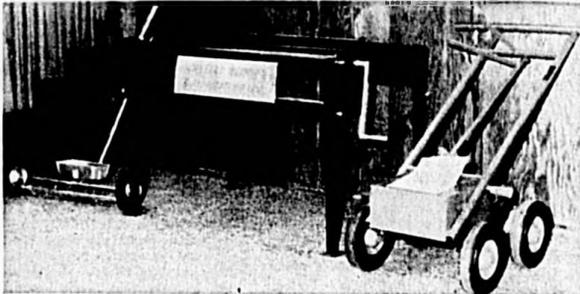
A MAGNETIC SWEEPER (left), a taping machine for fiberglass roofs (right) and a felt splitter, products of the Sanford Welding and Fabricating Co. are on display at the Industrial Show being held at the Civic Center. The magnetic sweeper can be used to pick up nails following, for example, a roofing job. (Herald Photo)
