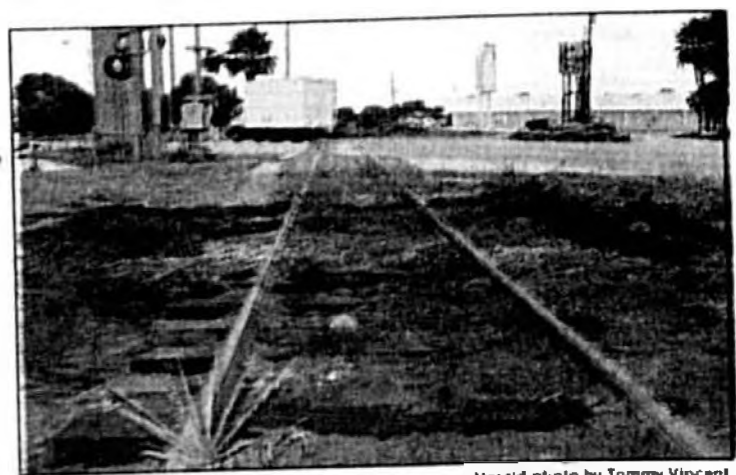
The Florida Department of Transportation announced the railroad crossing on U.S. Highway 17-92 will be rebuilt beginning Friday. The construction will necessitate total closure of French Avenue at the crossing beginning at 8 p.m. on Friday.
