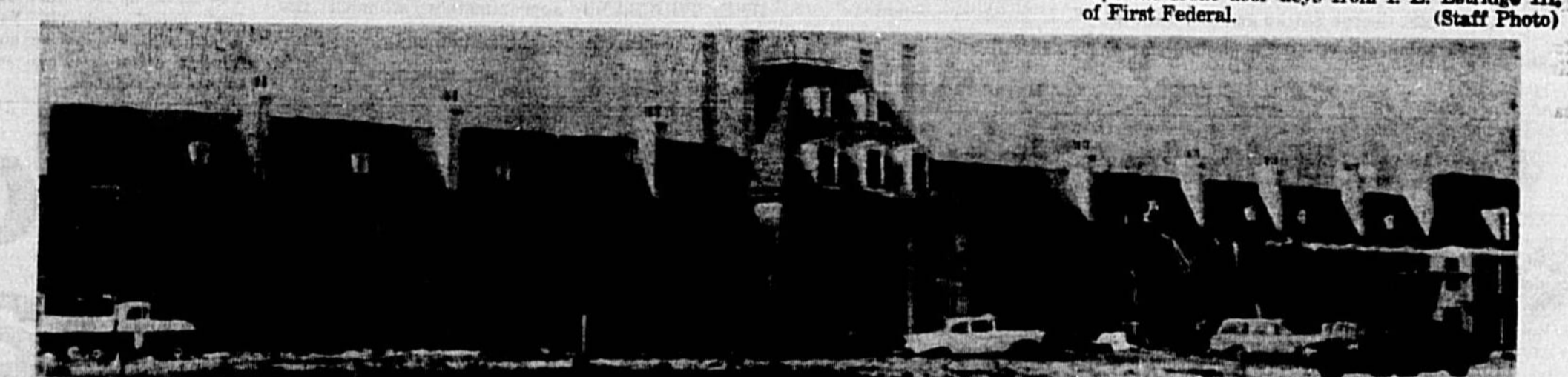
REGENCY APARTMENTS being constructed on SR 406 at Casselberry at the cost of $25 million will be one of the most elaborate in Central Florida. The 199-unit complex is in the French Renaissance style complete with garrets, spires, chimneys and red brick. The apartments range from one bedroom to townhouse and two swimming pools and other recreation facilities will be available for tenants. Clifford Wright is architect and Gardner Construction is contractor. (Photo by Jane Casselberry)
