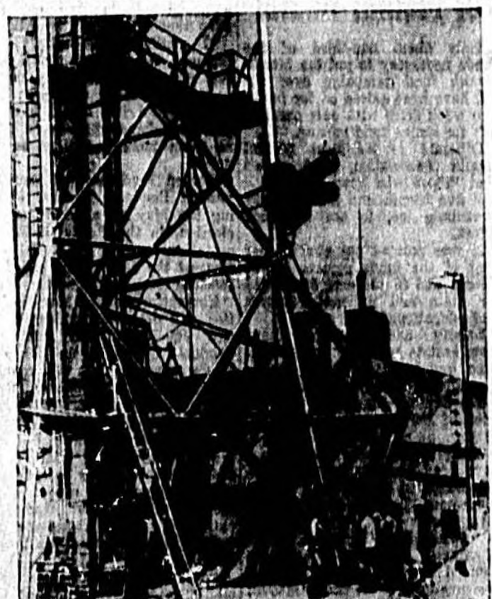
CIVIL DEFENSE OBSERVERS and newsmen inspect a concrete and steel-ribbed control bunker on Eniwetok Atoll in the Pacific, scene of the first airdrop of an American hydrogen bomb. The bunker, 20 miles from the target island of Namu, is designed to house scientists for several days in case the radiation should trap them. It is the closest point humans will be to the blast. A 300-foot high instrument tower stands at the left of the bunker. (International Radiophoto)
