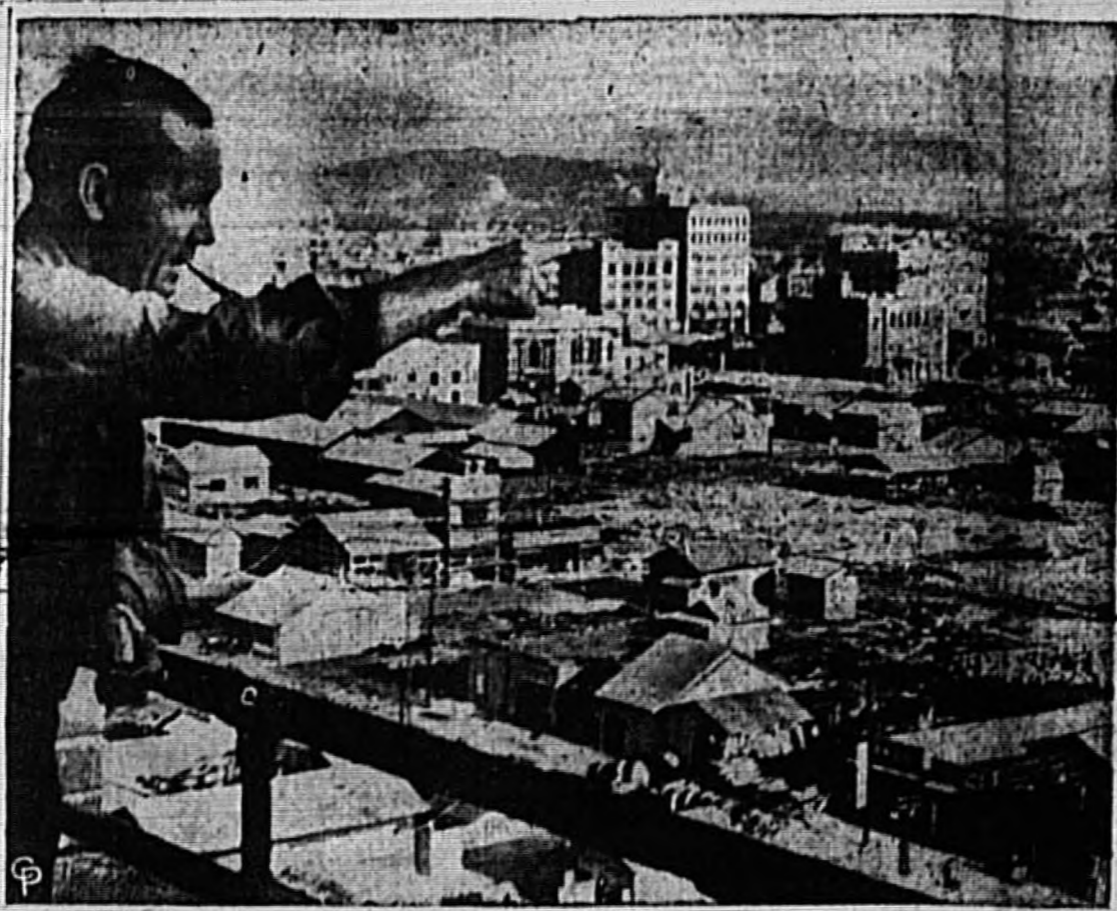
ALTHOUGH THERE ARE STILL MANY GAPING AREAS TO BE FILLED, Hiroshima, Japan, first target of an atomic bomb has made notable progress in rebuilding itself in the two years that have elapsed since the great blast in this Japanese city ushered in the atomic era. More than 50,000 new houses have sprung up from the city's rubble and more are going up every day. Long after the scars of the A-bomb have been obliterated, Hiroshima will be remembered as the unrelenting place of this new power. Photo from Look Magazine.
