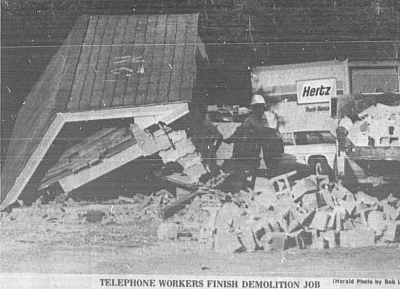
TELEPHONE WORKERS FINISH DEMOLITION JOB (Herald Photo by Bob Lloyd)
