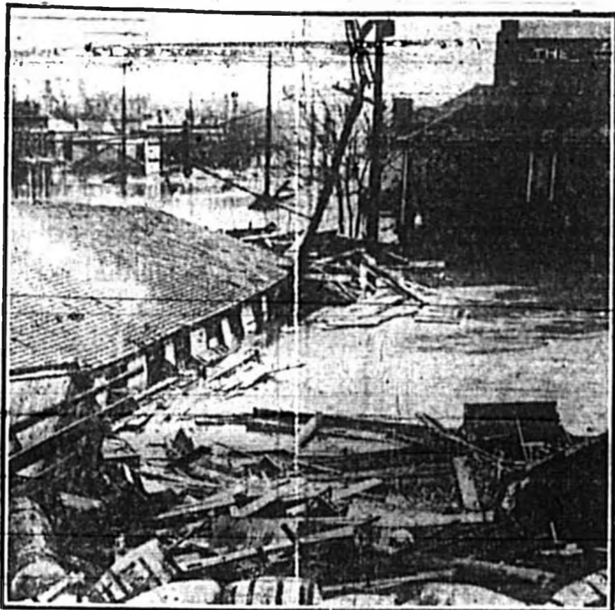
Photo copyright 1913 by American Press Association Tons and tons of debris were swept along with the rushing water. This wreckage collected against bridges and houses, forming dams which still further increased the height of the flood.
