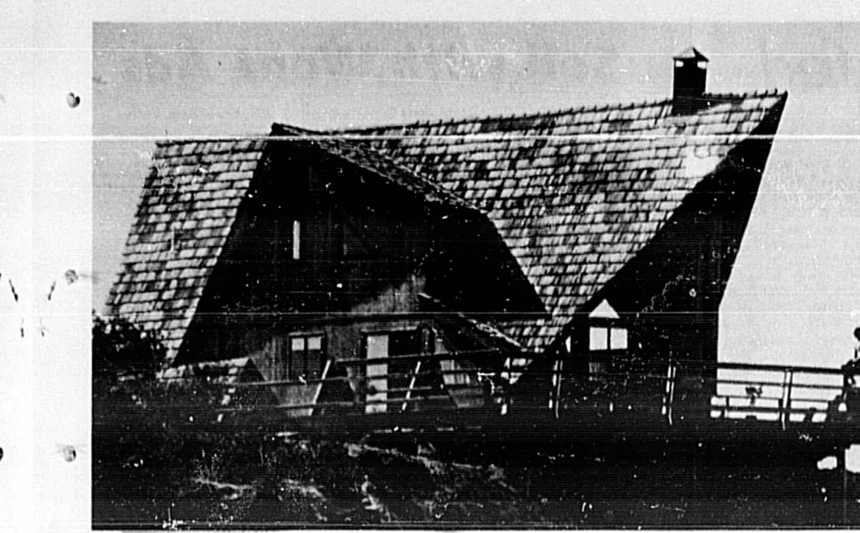
BOLD IMPRESSION — The roof of a modified A-frame house, rising 30 feet to the gabled peak, distinguishes this new house. Adding further emphasis to the roof appeal is the covering of heavy textured shakes. Note also the slanting V shape of the roof as it slopes toward a deck extending over a hill.
