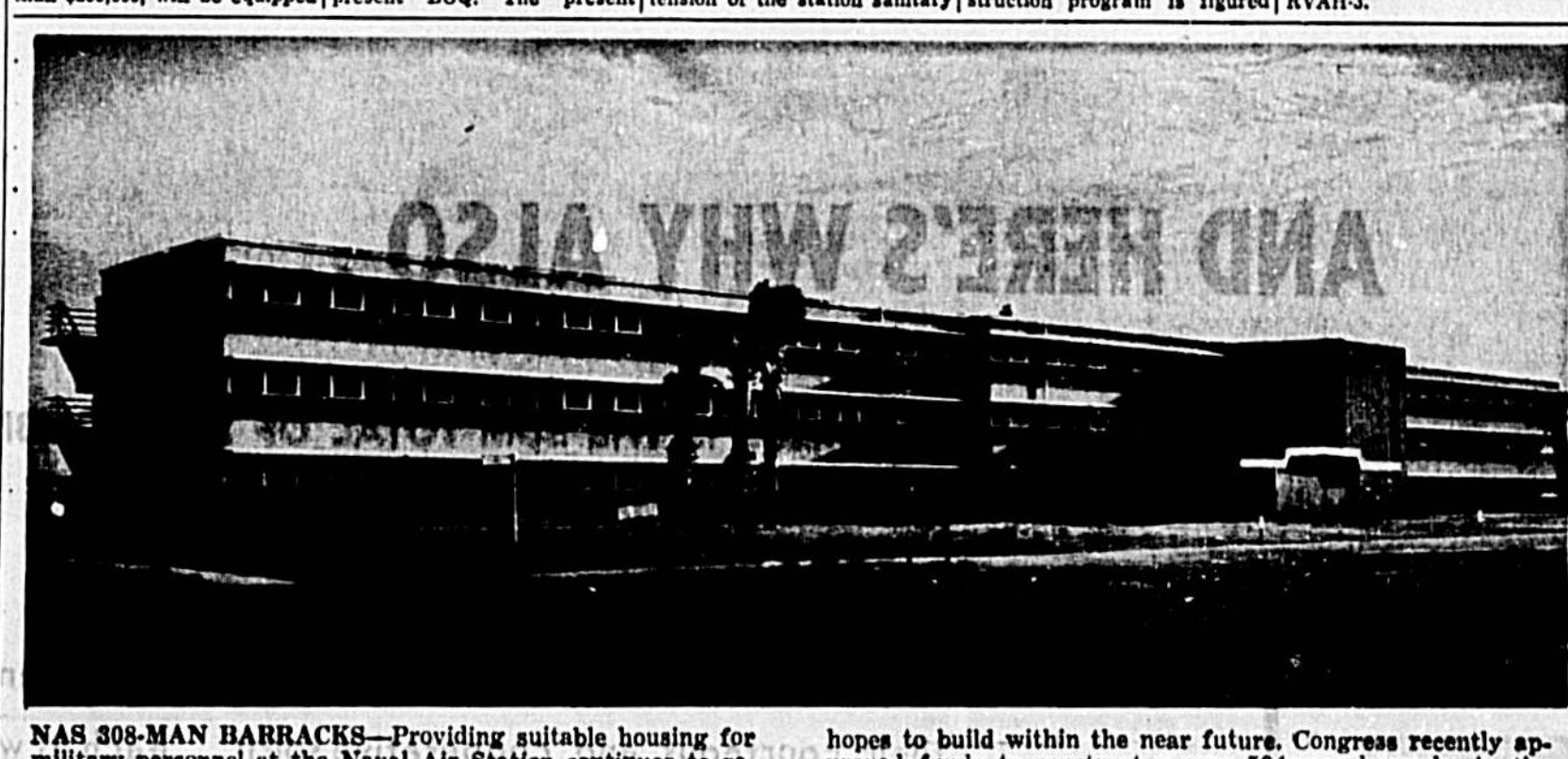
NAB 308-MAN BARRACKS —Providing suitable housing for military personnel at the Naval Air Station continues to receive top priority in the base construction program. This 308-man air conditioned barracks is the first of five the station hopes to build within the near future. Congress recently approved funds to construct a new 500-man barracks in the same vicinity as this one. (Official Navy Photo)
