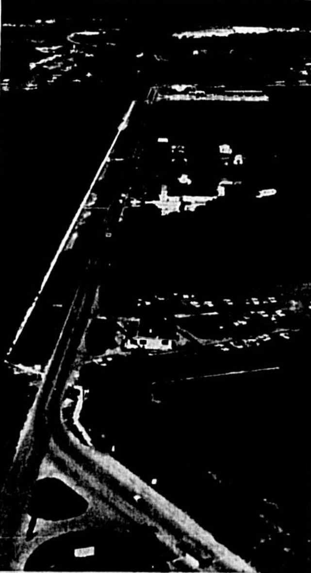
SAFETY SIDEWALK—Seminole County in cooperation with the Naval Air Station this summer installed a sidewalk between the station and Sanford Avenue along Onora Road. The station, concerned about pedestrians on Onora during morning and afternoon rush hour traffic, had been interested in the project for a number of years. The Navy purchased some $2,000 in materials, and the county did the work.
