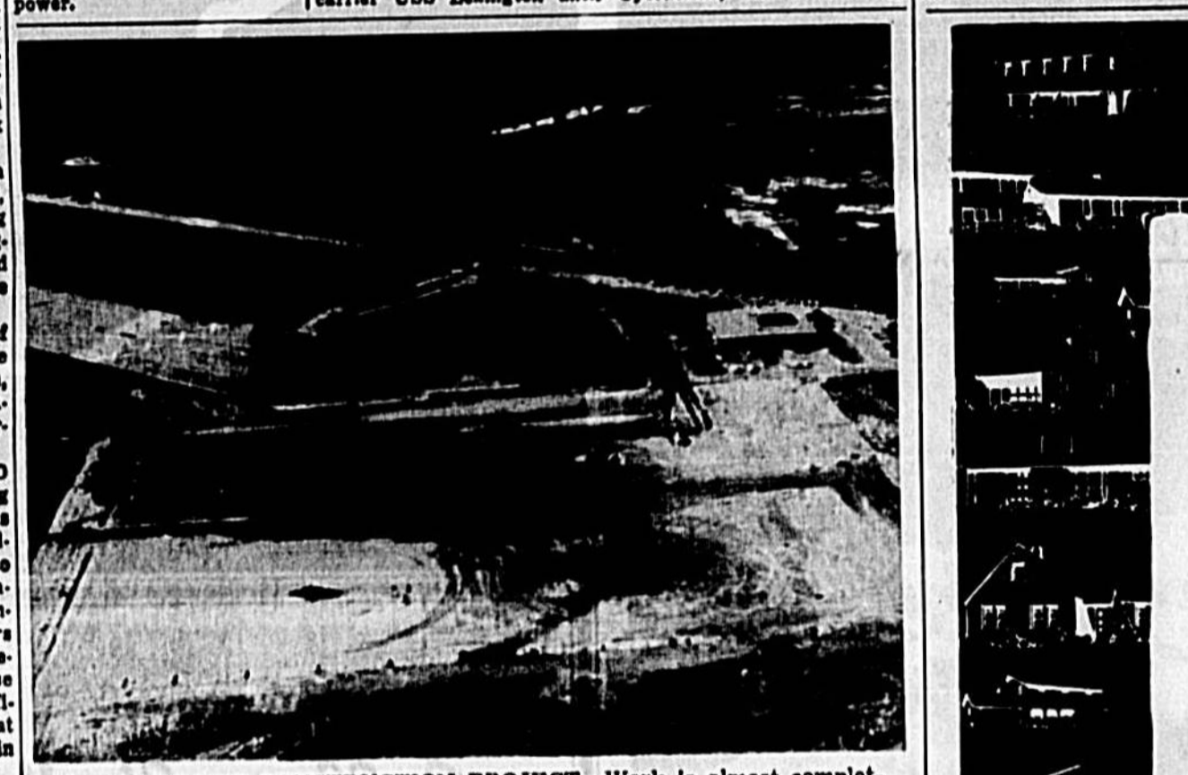
LARGEST NAS CONSTRUCTION PROJECT —Work is almost completed on a new aircraft parking area that will normally accommodate 16 RA-5C Vigilante jets at Sanford Naval Air Station. This $524,000 project is the largest to be launched during the current year at the base. The station Avionics Building can be seen at right center. A large hangar and an aircraft control tower is expected to be constructed just left of the building in the near future. Lake Golden is in upper left background.
