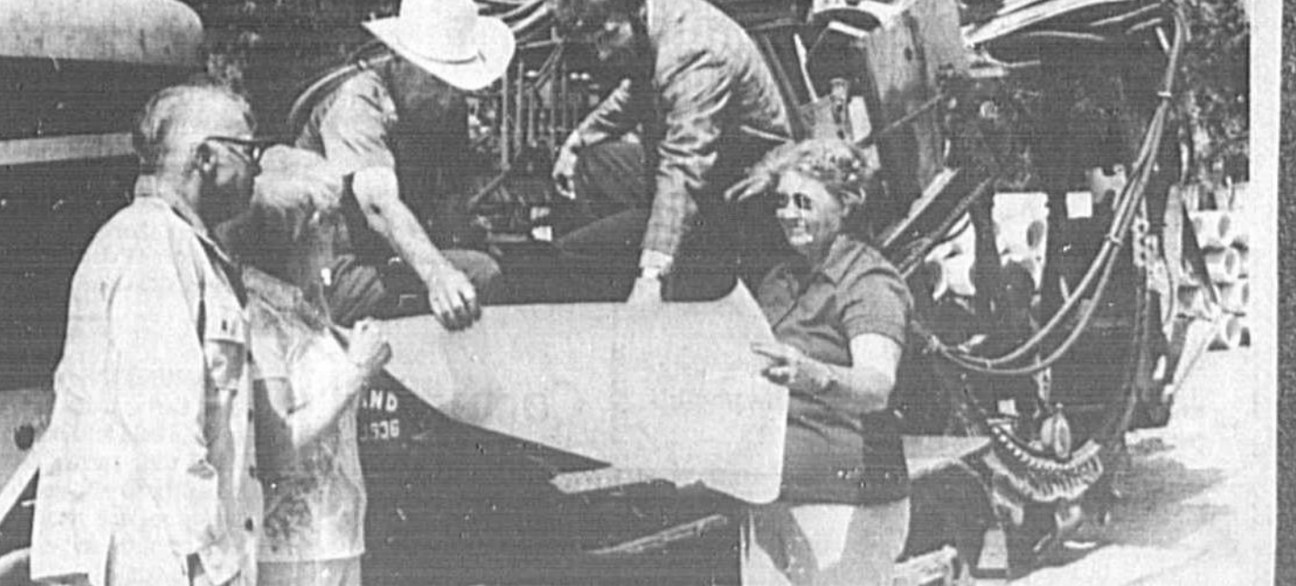
Work begins on $600,000 in Lake Mary's water system improvements financed through federal grants and loans. With W. B. Chisholm, superintendent of E. N. Murray Construction Co. contractors, (center) are Councilmen Cliff Nelson and DeLores Lash (left) and Mayor Walter Sorenson and Councilman Lillian Griffin.
