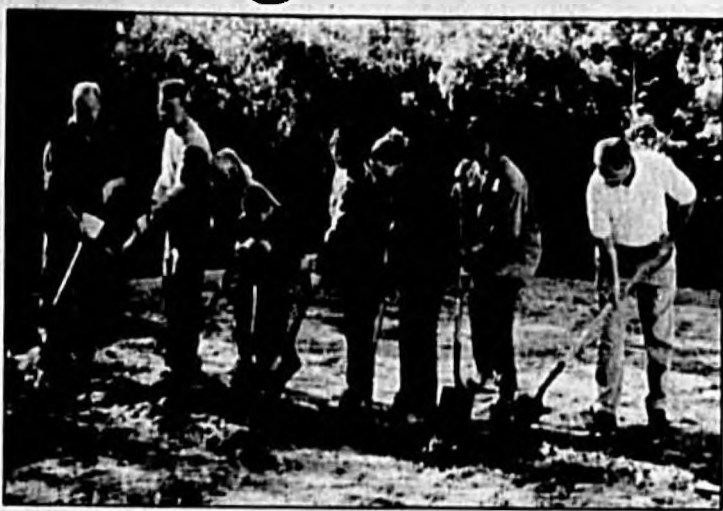
Photo submitted to the Herald Members of the Habitat for Humanity in Seminole County break ground on the organization's 50th house. Seminole Habitat, which recently celebrated its 10 year anniversary, plans to build 50 more houses in the next five years.
