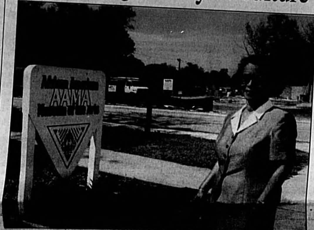
Irene D. Johnson stands in front of the Phase I construction occurring at the African American Museum of the Arts in DeLand. Once completed, the facility will include a cultural park and amphitheater. Herald photo by Tommy Vincent
