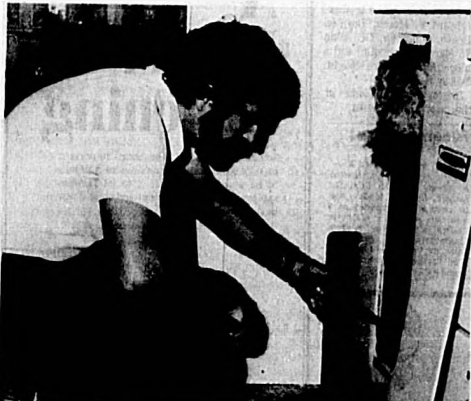
Tim Dell, Florida Power & Light Co. energy auditor, adjusts a water-heater thermostat to 120 degrees, sufficient for a family without a dishwasher. Installers normally set the thermostats on water heaters at 150 degrees.
