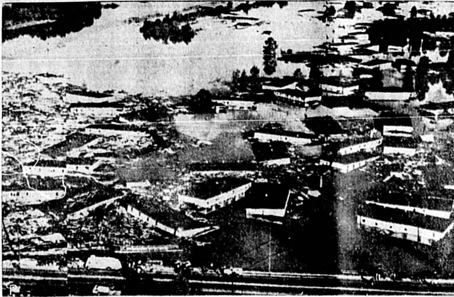
CRUMPLED TWO-STORY APARTMENTS of the war-built town of Vanport, Ore., lie jammed together in tangled piles where flood waters that poured into the river burst. Lower stories of the frame buildings are under possibly scores of victims who lost their lives in the deluge. fled frantically to escape the flood.
