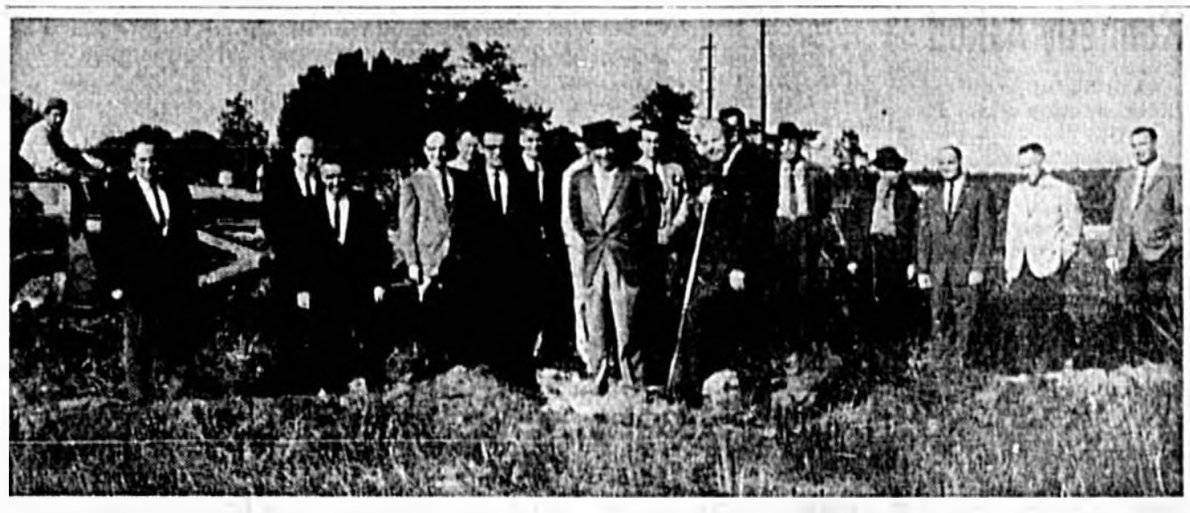
GROUND-BREAKING ceremonies took place this morning at 10 a. m. at the new industrial site of the Del Mar Cabinet Industries Corporation of Atlanta. Present at the new project were Sanford-Seminole Development President Cliff McKibbin officiating, several representatives of the company, as well as Sanford businessmen and local officials. The Del Mar project is the first authorized in the state under the new Small Business Administration. (Herald Photo)
