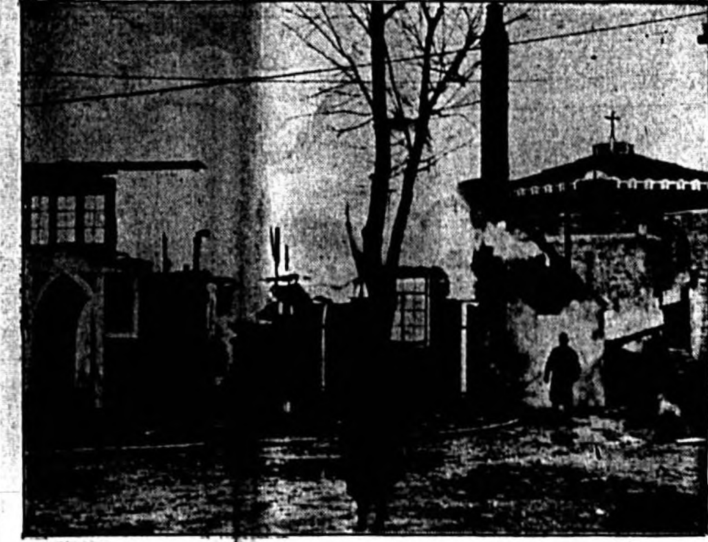
Father Charles E. Coughlin's original Shrine of the Little Flower at Royal Oak, Mich., stands in ruins after a fire attributed to faulty wiring. Damage was estimated at $30,000. In the background at the right can be seen the dome of the famous radio priest's new $500,000 church which escaped damage. (Associated Press Photo)
