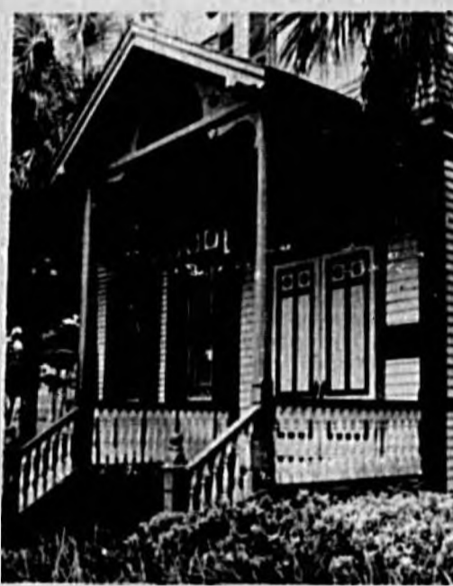
Front porch of DeLand Hall
