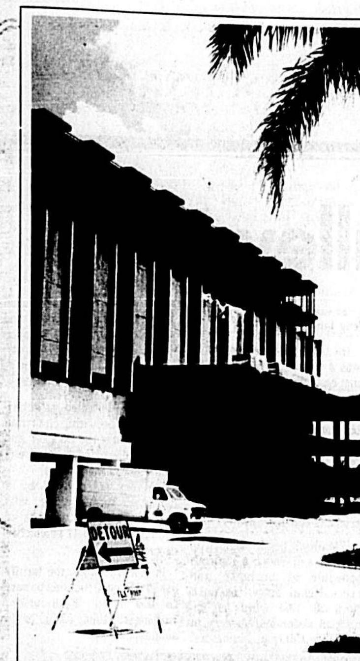
Construction underway at Florida Hospital. Two floors are being added.
