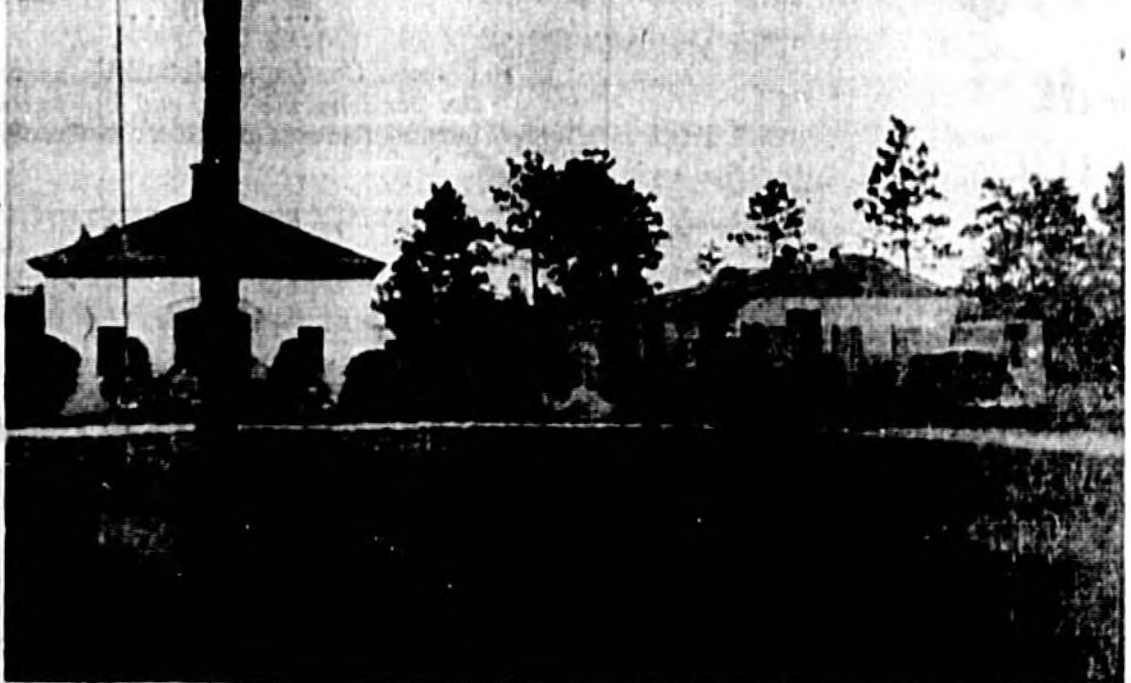
NEW SCHOOL WING—A new wing is in the program of being added to the St. Luke's Christian Day School at Slavia at a cost of about $25,000, according to the Rev. G. M. Tuby, pastor of the Lutheran parish. The new building (right) will include two classrooms, a library, office and a small theater room. A loggia will attach it to the rest of the school building. The school originally was planned to include three wings. Two wings include two classrooms and the auditorium. E. L. Bellhorn is principal of the school. Work is being done by Rhoads-Watson, Inc., Winter Park. Most children in the area attend the school, but any child may attend if he is provided his own transportation, according to the Rev. Mr. Tuby. (Staff Photo)
