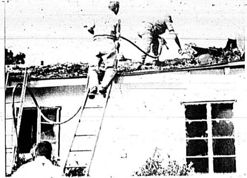
WRECKAGE STREWN ATOP HOUSE IN DEBARY ... Firemen, volunteers probe for blame
