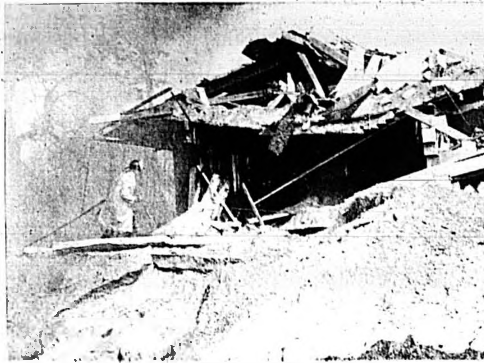
DAMAGED HOME PROBED BY FIREFMEN ... Shell Road home, one of two destroyed
