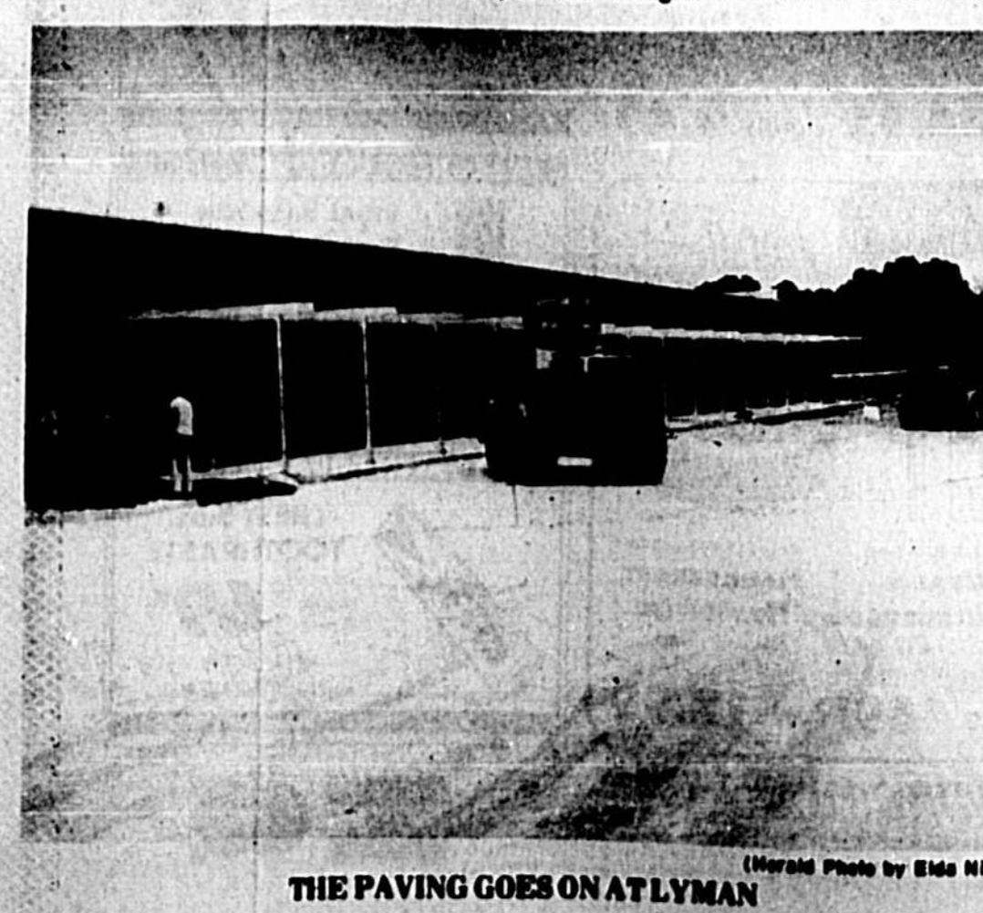
THE PAVING GOES ON AT LYMAN
