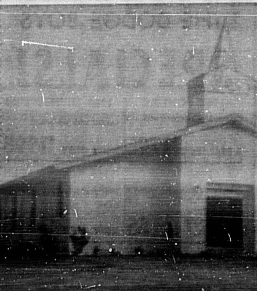
THIS NEW sanctuary of the First Pentecostal Church at Longwood, built at a cost of $55,000, was dedicated recently in special services conducted by the Florida District Superintendent of United Pentecostal Church, Rev. William Connell of Ocala. Rev. Luther C. State home mission director, preached the dedication sermon. Rev. W. S. Craig Section 2 presbyter, gave the prayer and local pastor is Rev. Ruth Grant. The church opened 11 years ago with 15 enrolled in the Sunday School which has grown to 110.
