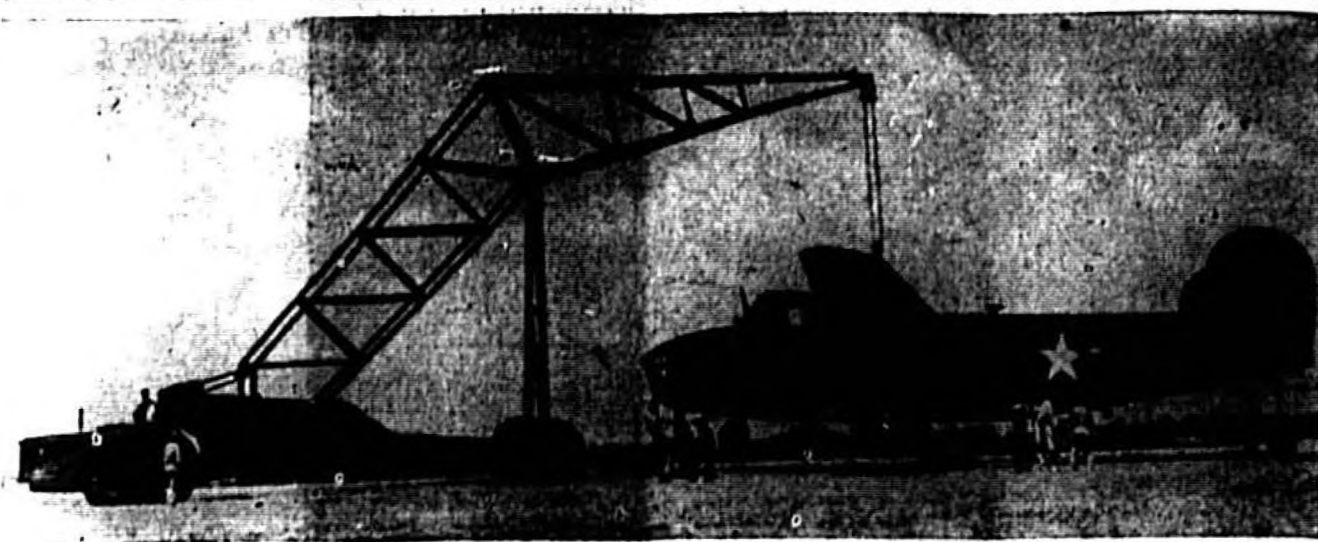
This huge new wrecking crane, a mobile unit, developed by the U. S. Army Air Corps, is shown lifting a heavy B-24 bomber plane during a clearing operation at Patterson Field, Ohio. An undisclosed number of these big hoists are in production at present and will be used for clearing runways of damaged or wrecked aircraft. Flying fields, temporarily out of commission because of wrecked planes, will be made fit for use in a short period of time by having equipment of this type on hand. This is a photograph. (Central Press)
