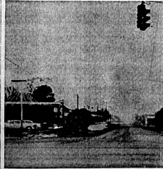
TAKING SHAPE is the four-lane section of First St. which is being widened from French Ave. to the intersection of Interstate 4. The picture shows the width of the $600,000 project which will give Sanford adequate access to the new expressway when it is completed. (Herald Photo)
