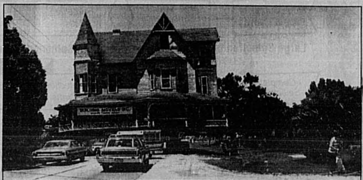
Moving Day for the Bradlee House formerly of Altamonte Springs, FL.
