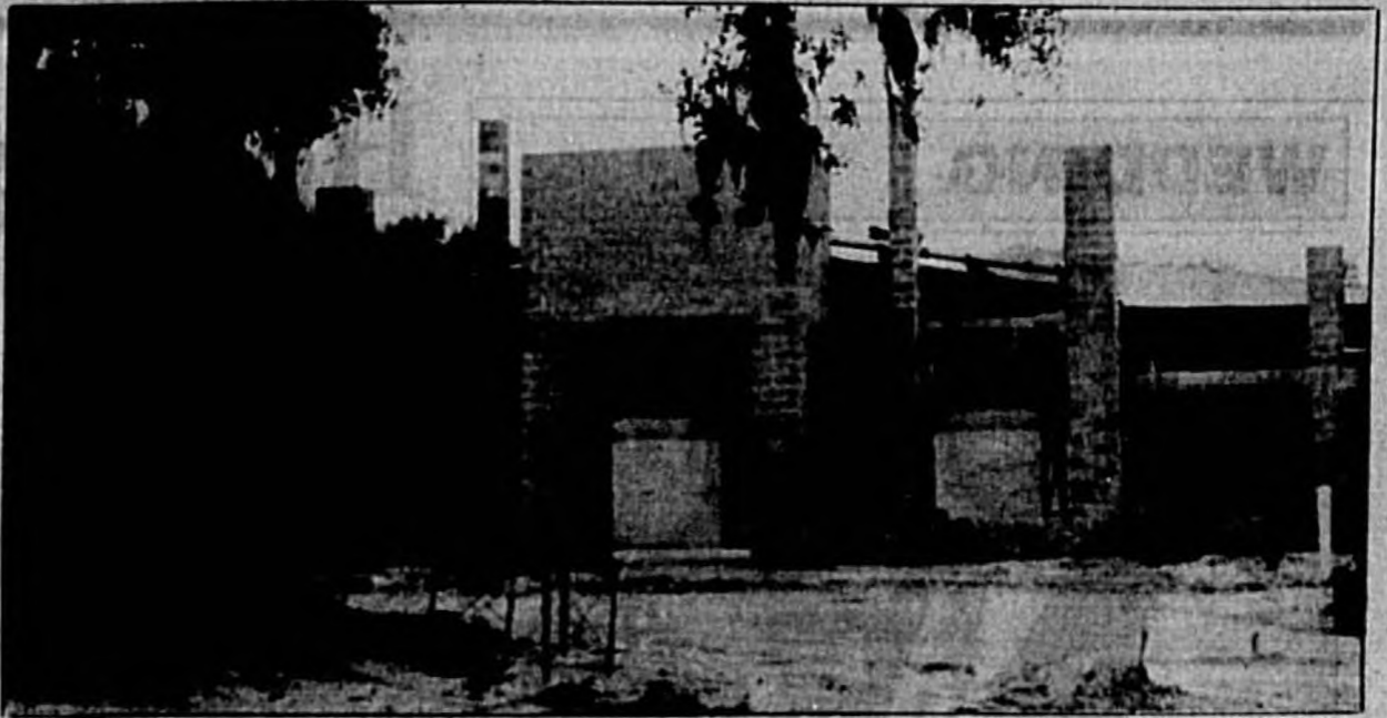
The Seminole YMCA Family Center is undergoing a 19,000-square-foot expansion.
