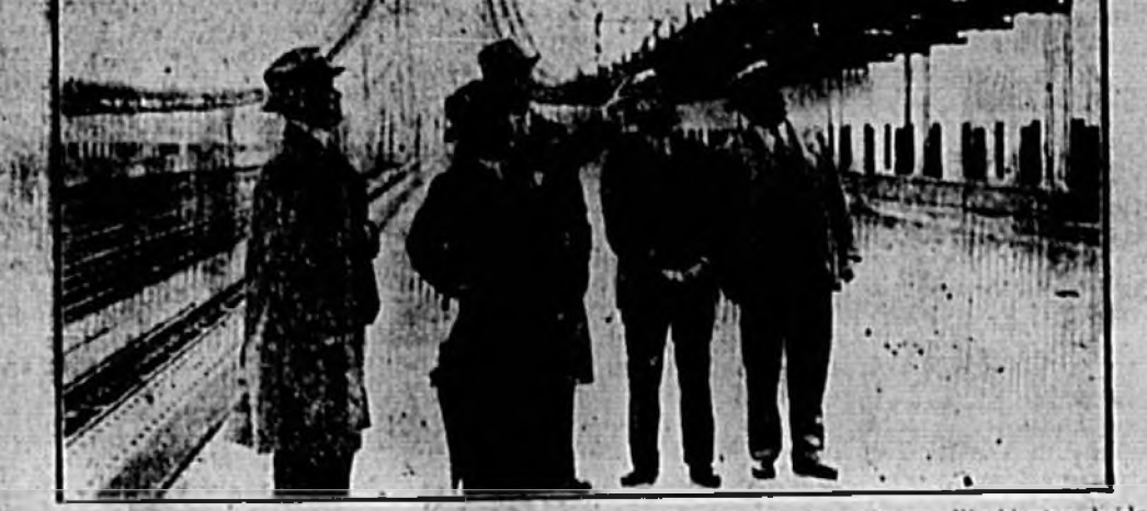
Here you see a group of bankers on an official inspection of the giant George Washington bridge over the Hudson River. Photo shows John F. Galvin, chairman of the New York Port Authority; George de B. Keimig; N. B. Seeley, and Dr. L. Norwood.
