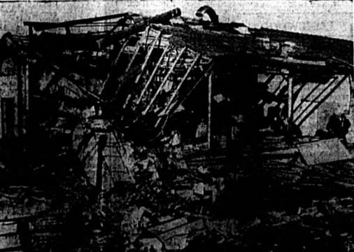
Firemen search rulns of the National Magnesium Co. plant in Newark, N. J., after the building was destroyed by an explosion, killing two. The plant manufactured magnesium powder for the army and navy. New dust collector device was blamed for igniting the powder.
