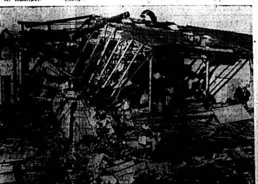
Firemen search ruins of the National Magnesium Co. plant in Newark, N. J., after the building was destroyed by an explosion, killing two. The plant manufactured magnesium powder for the army and navy. New dust collector device was blamed for igniting the powder.
