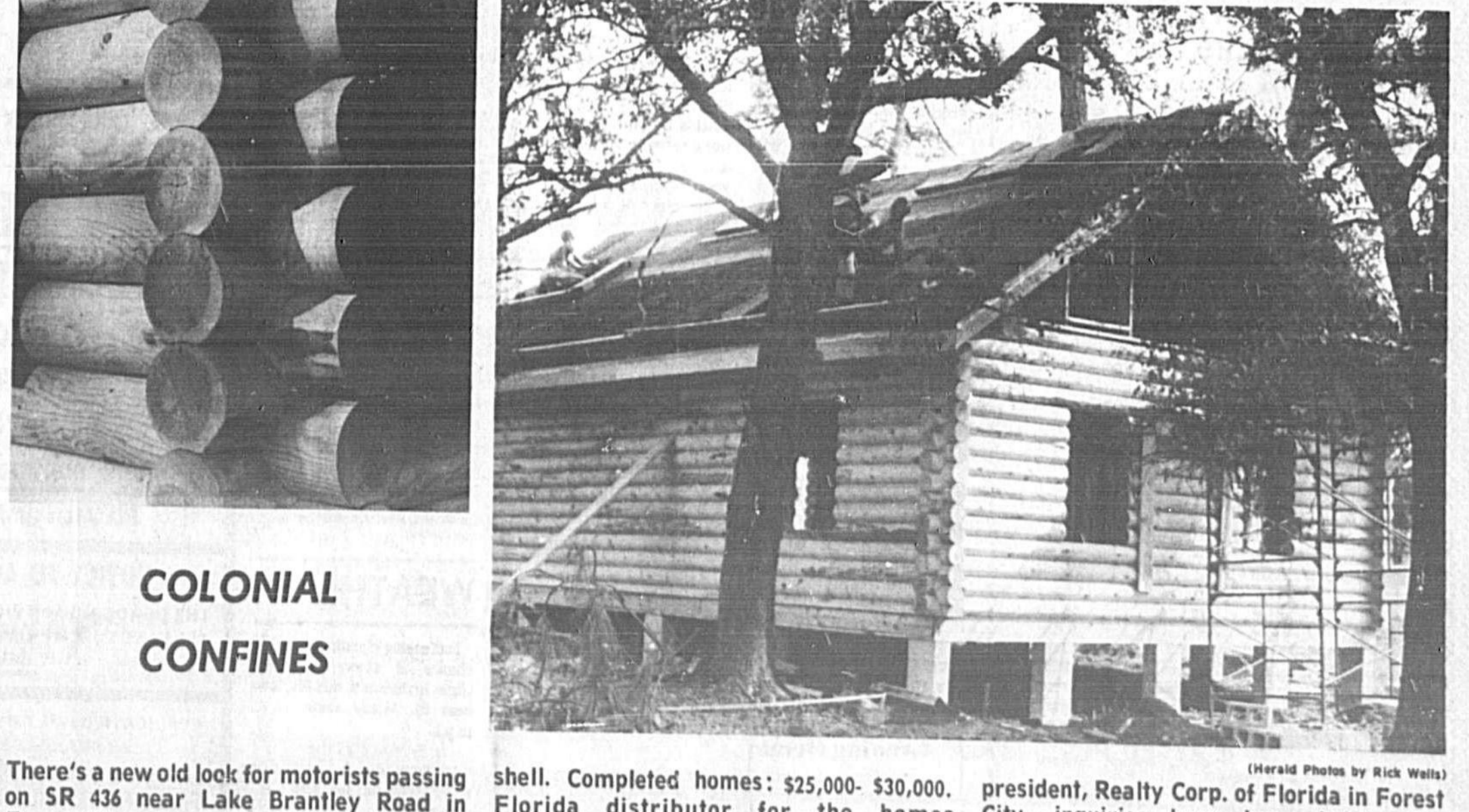
COLONIAL CONFINES. There's a new old look for motorists passing on SR 436 near Lake Brantley Road in Forest City: a 24x36 log cabin. Built from a kit reminiscent of the Lincoln Logs of years past. Cost of package is $2,000 for the smallest unit and $10,000 for the largest shell. Completed homes: $25,000-$30,000. Florida distributor for the homes Gatliffburg by Log Cabins Inc., of Gatliffburg, Tenn., is All-American Log Cabins. According to Wally McGuff, factory representative, and John H. Wright, president, Realty Corp. of Florida in Forest City, inquiries have been brisk. Explanation says McGuff: 25-35 per cent savings over conventional construction and a "grassroots surge back to the things of our forefathers."
