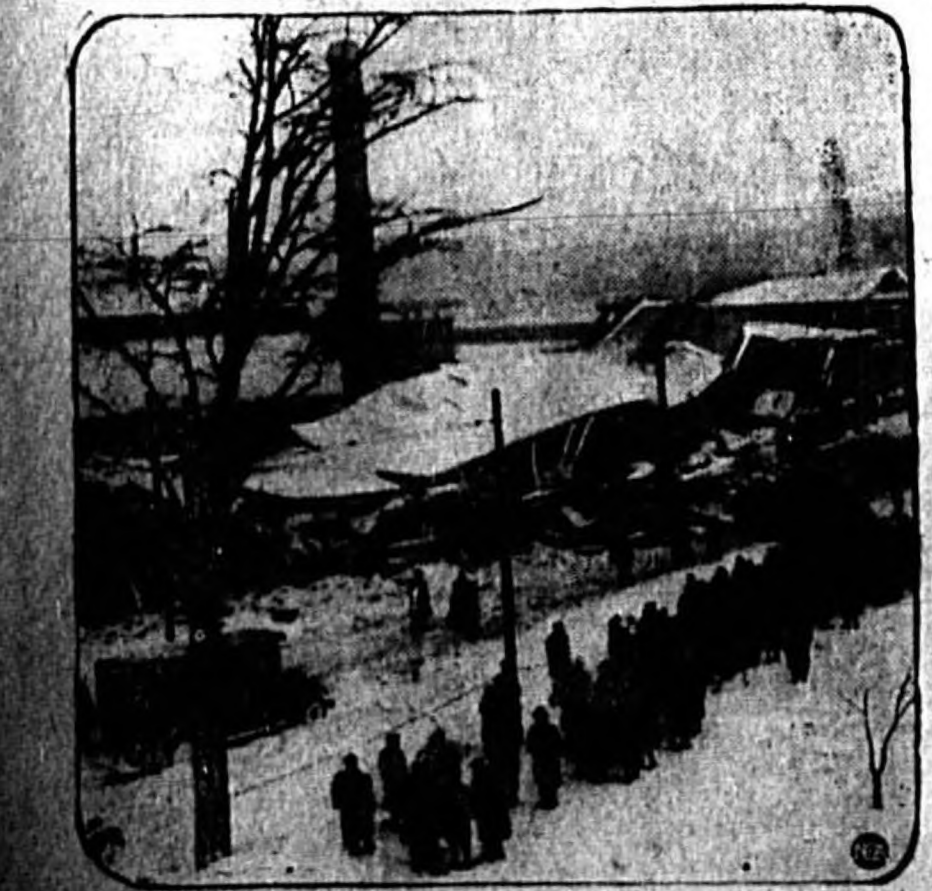
In ruins of the collapsed North & Judd Manufacturing Co. foundry, New Britain, Conn., shown above, 20 persons were buried and eight lost their lives. Snow piled up on the roof until it gave away.
