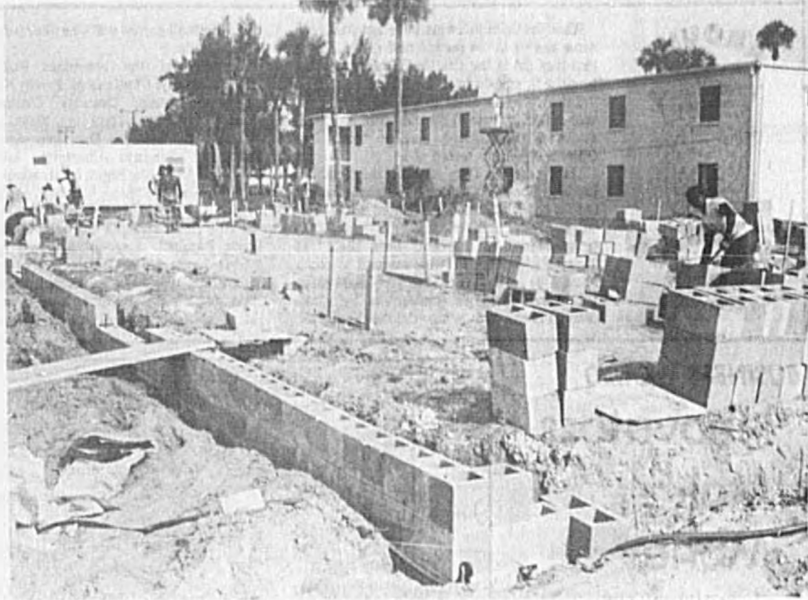
Foundation Is Being Laid On New Data Center
