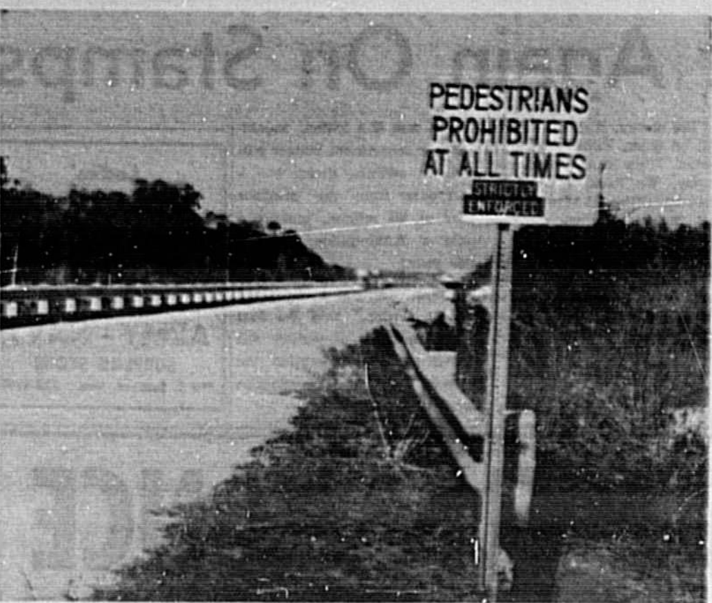
GHOST WATCHERS beware Snow Hill Road bridge is off limits for pedestrians and parking. (Liza Baker Photo)
