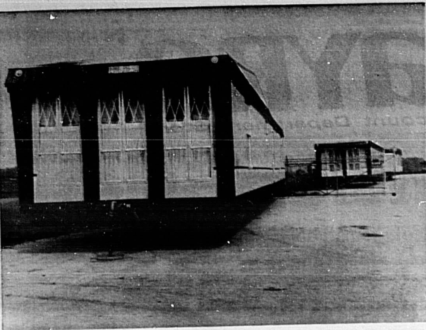
WINCHESTER HOMES are on display at the former H. L. Hunt canning plant on Sanford Avenue in Sanford. Manufactured at Winfield, Ala., by TUFTCO, parent company of Winchester, these models soon will be constructed here by an estimated 800 employees trained to staff 19 assembly lines. Production is expected to start here by November. (Bill Scott Photo)
