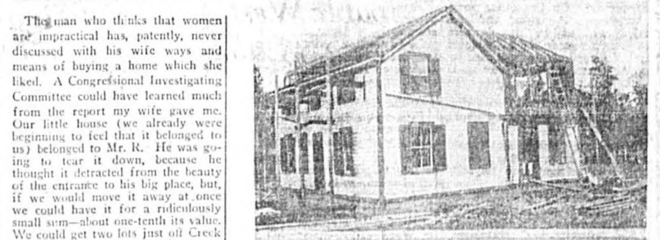
Above: The House As It Is Now. Below: When Reconstruction Started.
