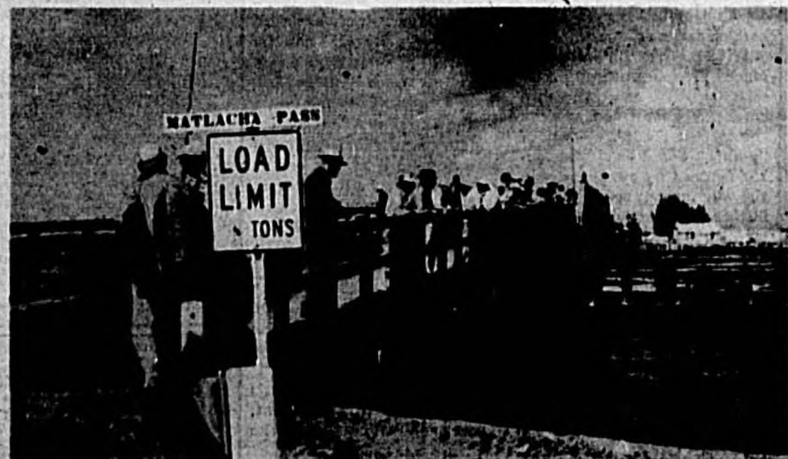
FISHERMEN CROWD Pine Island Bridge at Matlacha Pass, west of the drawbridge section.
