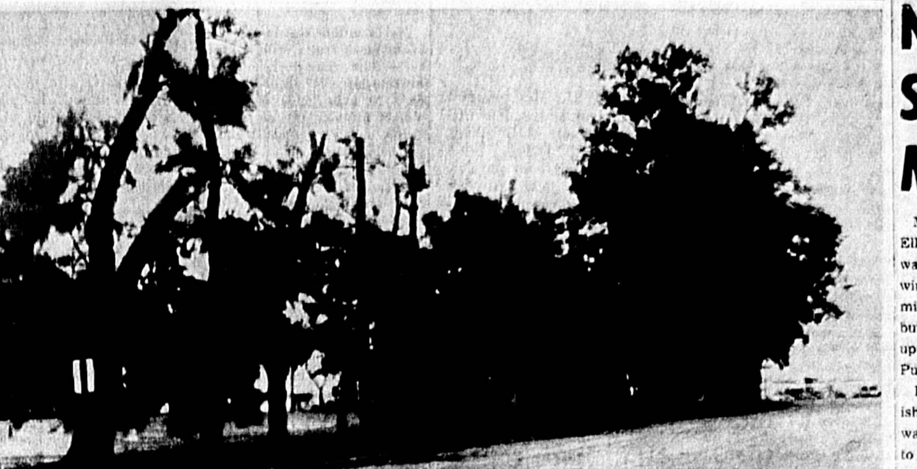
PINE TREES on Palmetto Avenue across from the postoffice were topped off by the Florida Power and Light Company in the first step of the operation to make way for the installation of feeder power lines to the new marina-motel complex. Work was halted temporarily at the "request" of City Manager W. E. Knowles until all equipment necessary to remove the trees completely is present on the site. Work is expected to resume Wednesday. (Herald Photo)
